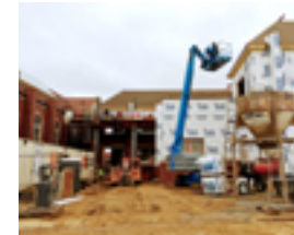
Construction continues on the new Welcome Center
